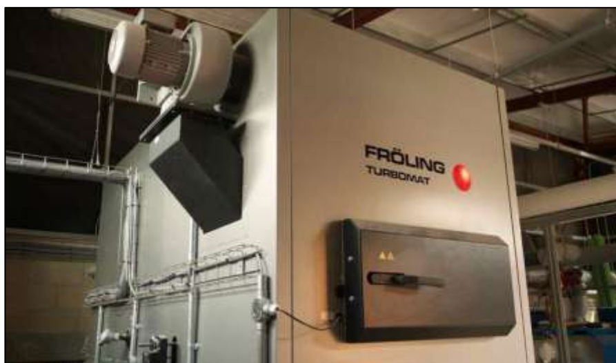
The College's biomass boiler, which was installed in 2011, heats, via a district heating system, almost all of our teaching rooms, the library, support services building and a number of our leisure and recreation facilities.
